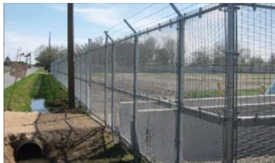
Photo: Wirewall by Riverdale
